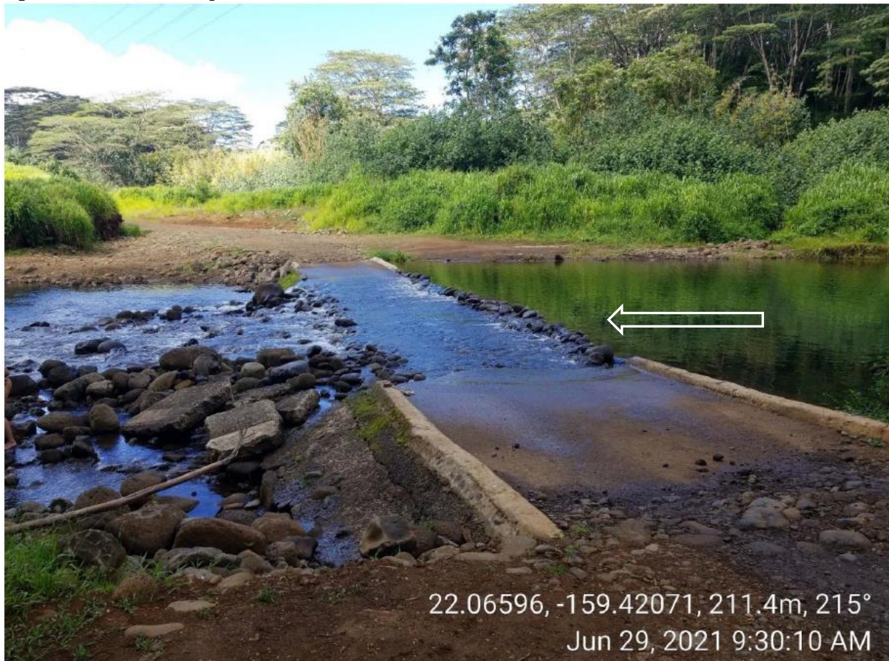
Figure 2: Site Photo looking south.
